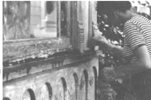
With that job out of the way, **LiquidWood** can now be applied to the deteriorated wood. One part of **LiquidWood A** is thoroughly mixed with one part **LiquidWood B**. After waiting about 5 to 10 minutes after mixing, the A/B blend is then applied directly to the deteriorated wood where it is absorbed like water is absorbed into a sponge. It should be reapplied until the wood is saturated and will no longer absorb it.
