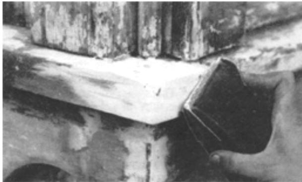
If restoring a window sash, or any structures where two pieces of wood may tend to flex, a dowel pin can be inserted where the two pieces join for added fastening.
