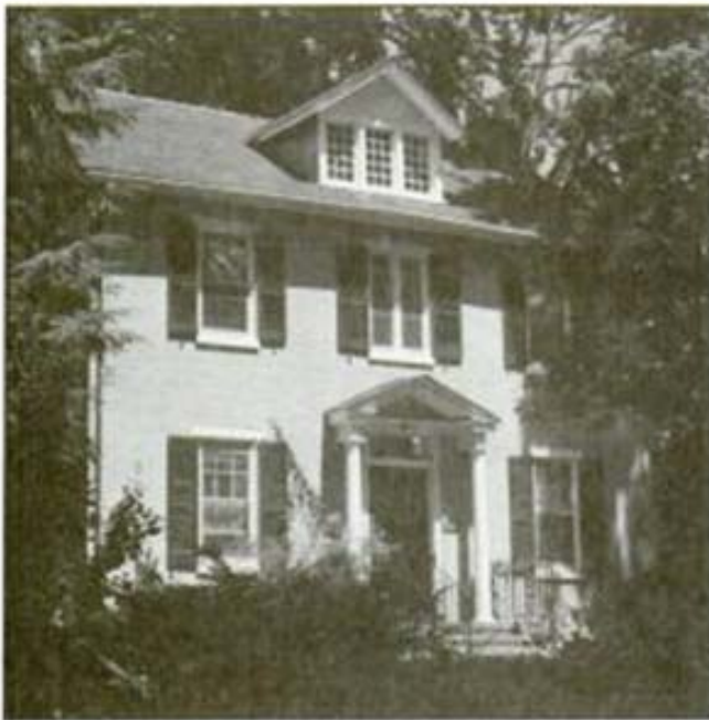
A brick house can be sensitively painted. This building has been successfully painted in a Georgian color scheme.
