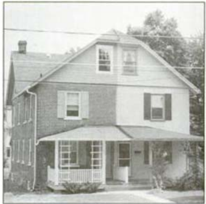
Then again, painting brick can create an eyesore — as evidenced by this schizoprenic house.
