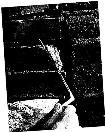
Before you can repoint, you have to determine the right mortar mix to match the existing mortar's color and the hardness of the brick.
