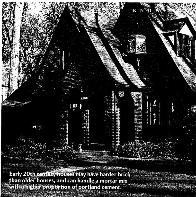
Early 20th century houses may have harder brick than older houses, and can handle a mortar mix with a higher proportion of portland cement.
