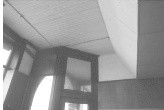
One technique that can be used to achieve positive results with less cost is to remove only the front portion of the suspended ceiling.
